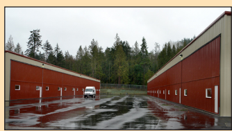
Port tenant 48° North built new hangars at Anacortes Airport.
