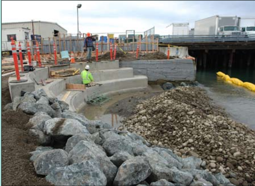
IMPROVED PUBLIC ACCESS: Among elements of an "O" Avenue beach project adjacent to Port of Anacortes facilities on the Guemes Channel is this stairway/seating section leading from street level to the beach. To the east of this section are street improvements including sidewalks and surface tiles that allow water to permeate through into the earth. This section of public beach and street are located just to the north of Port tenant Puget Sound Rope. Project elements also included removal of creosote coated pilings posted decades ago near water's edge. Completion of the work is anticipated in early December.
